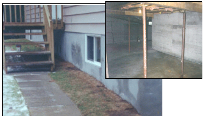
Figures 2 and 3: Current homes are typically built with underground concrete basements resulting in small windows and dark, damp, unhealthy living areas
