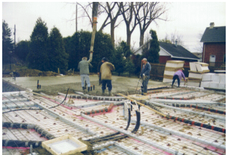
Figure 1: The LEGALETT slab contains a network of closed loop air ducts which circulate warm air from integral heat distribution boxes in the slab.
