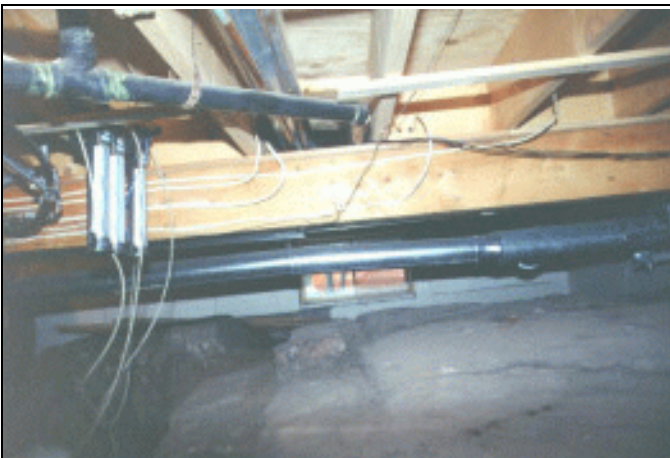
Figures 4: Basement built into rock
