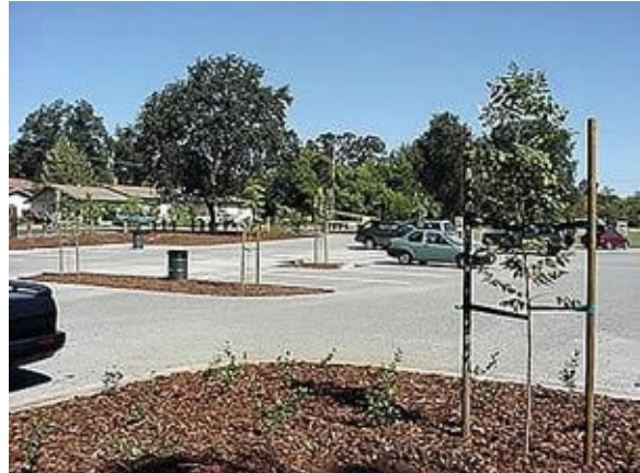
This parking lot installed in 2001 at Bannister Park, Fair Oaks, Calif., is the first in the state to use pervious concrete. The Sacramento Cool Communities program was a partner in the project, which used pervious concrete for stormwater management and to reduce the urban heat-island effect. In about 10 years, the trees will shade more than half the lot.
