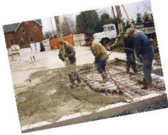
undergirding the perimeter of the slab. It is reinforced with steel rebar and is not frost-protected (there is such a thing as a frost-protected slab-on-grade but it is not done in Canada). The grade beam and slab are usually designed to "float" as a single unit above the frost line. As a result, it moves and cannot be used as a foundation for a home.
