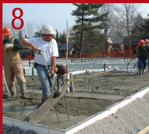
Place and Finish Concrete
