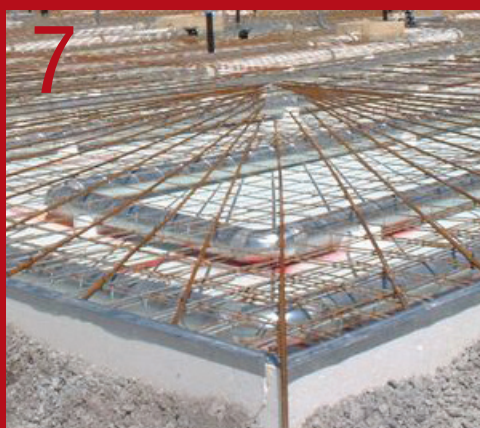
Install Final Reinforcement
