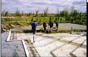
When the great Ontario ice storm of 1998 cut the power in this Cornwall home, it took a week for the home to drop from 72 degrees F to 67 degrees. The reason: the 2,300 sq. ft. LEGALETT system concrete slab beneath the house acted like a massive heat sink. The insulated slab held its heat and heated the home for days after the power was cut.
