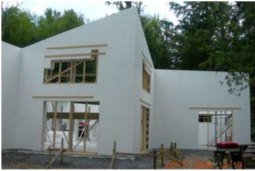
This modern cottage design incorporates the latest in building methods and materials. The Legalett air-heated "Slab on Grade" system was the perfect solution for heating this Upper New York State getaway built using Insulated Concrete Form walls.
