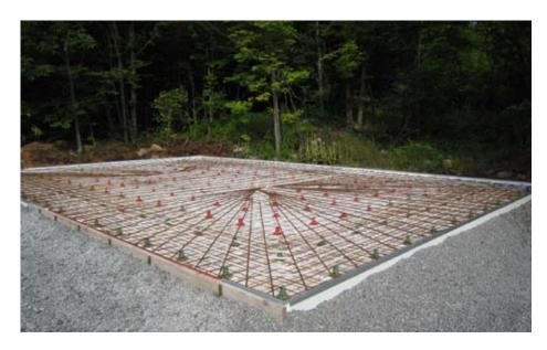
This 36' x 24' Legalett Frost Protected Slab was installed to accommodate an unheated garage, following the property owner's residential construction, which also used Legalett slab technology (See Profile 6024).
