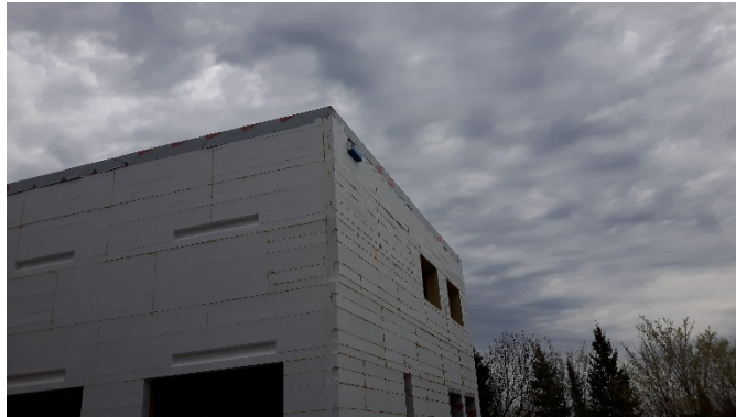
This image illustrates the corner placement of ThermalWall PH panels
