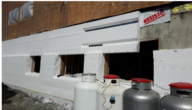
Studs removed for cutting around windows
