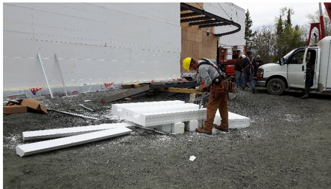
Panels are easily cut with a chainsaw
