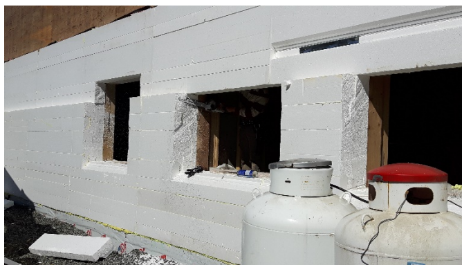
Trim openings easily with a chain saw
