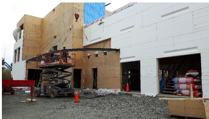
Installing an entry frame for a canopy
