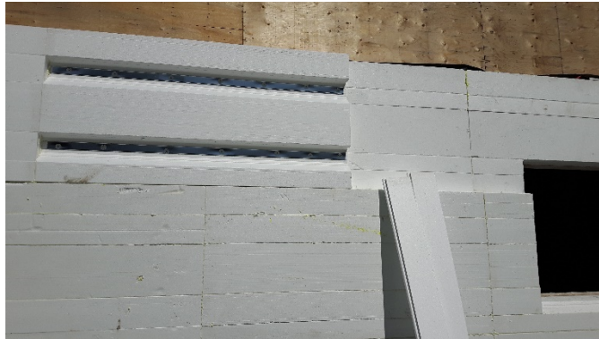
ThermalWall PH Panel is installed and ready for snap tracks
