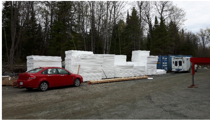
ThermalWall PH Panels delivered to site and ready for install
