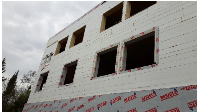
This image illustrates the installation of window flashing and build outs
