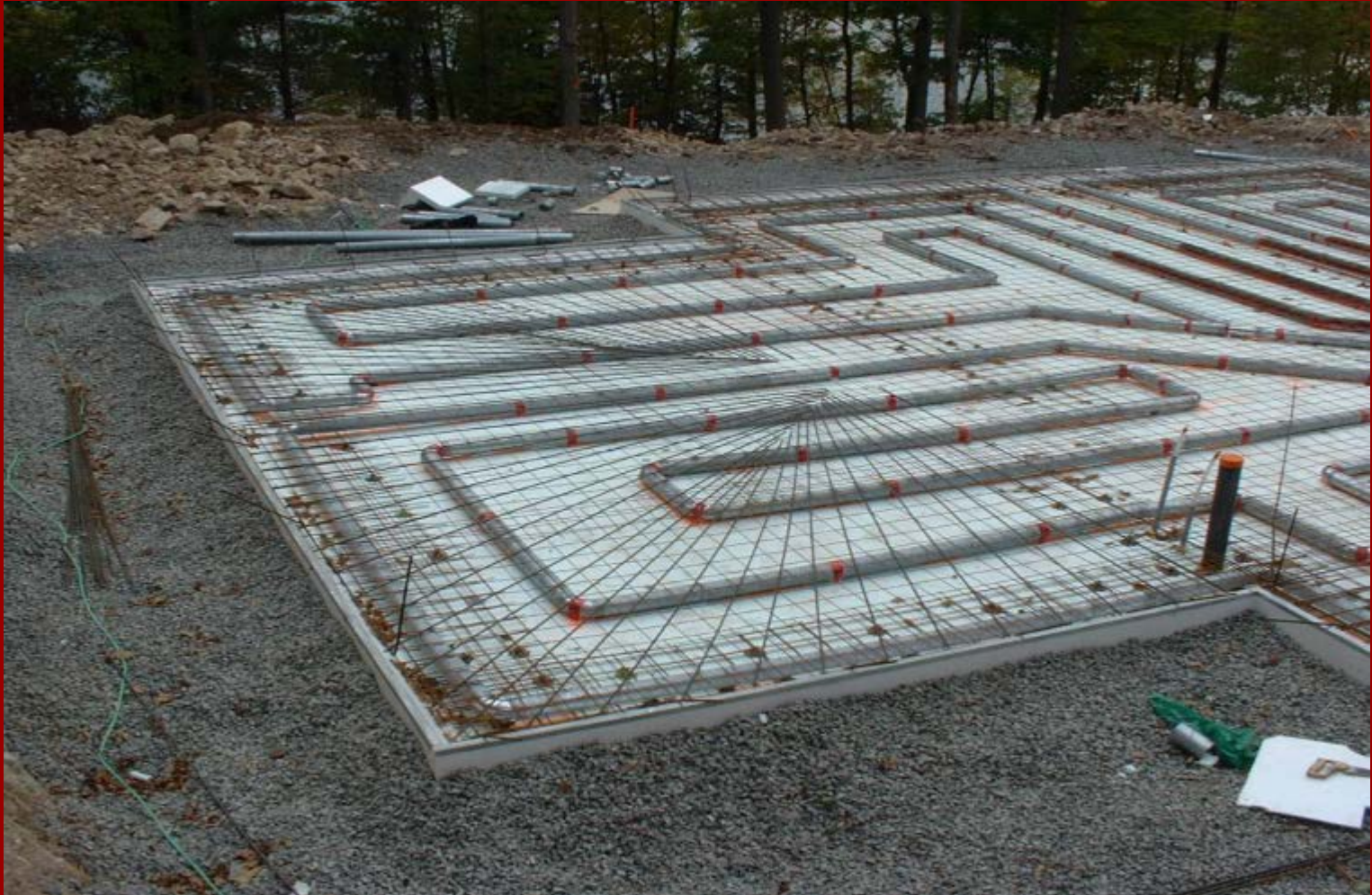
Frost Protected Shallow Foundation (FPSF)
