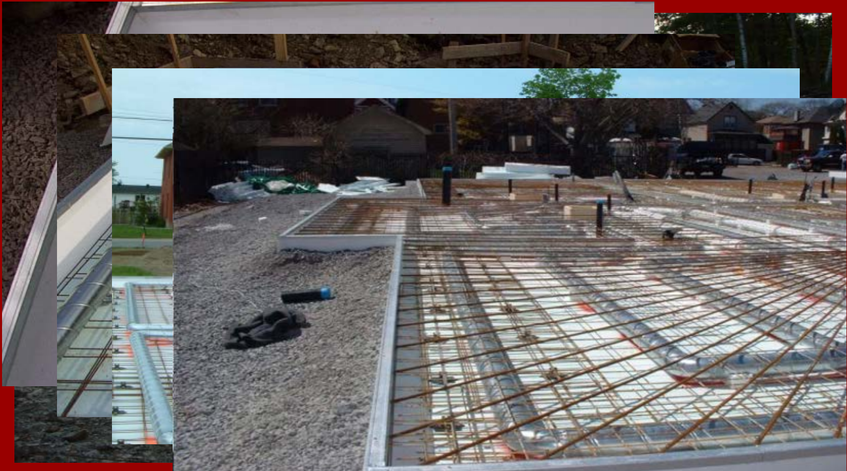
Install mesh, piping and piping insulation
